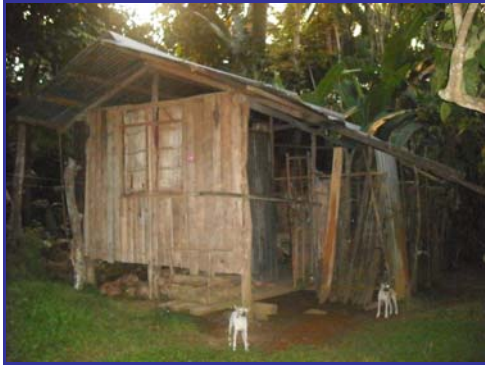
Front of the house—BEFORE
